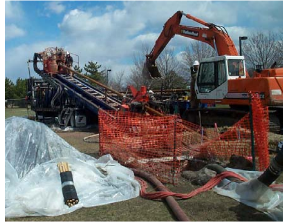
Figure 3.18 The directional drilling [75]
