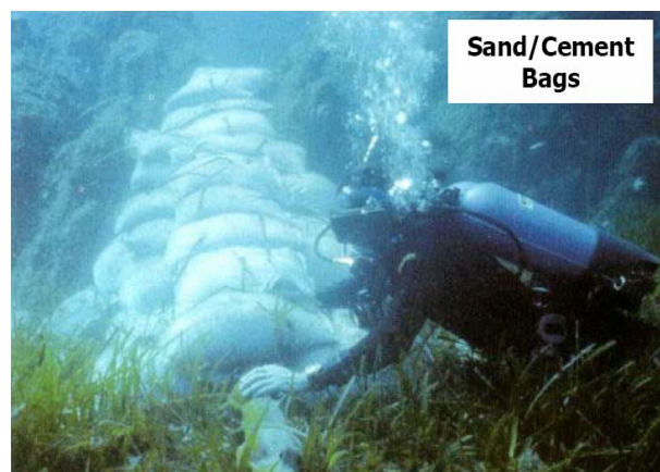
Figure 3.20 The sand/cement bags [67]
