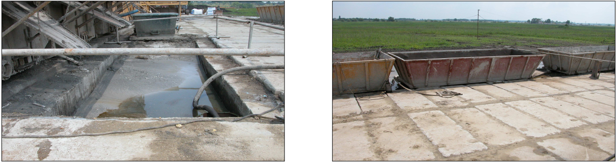
Figure 1.5: Sealed Concrete Pit (Left) and Collector Pits (Right)
