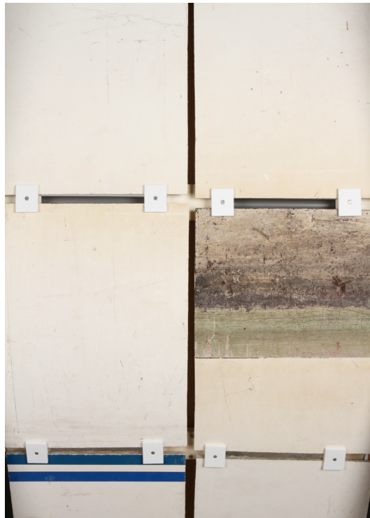
FIGURE 10 BOAT HULL PANELS IN A MOCK-UP OF FAÇADE, PHOTO BY M. BILOW, PROJECT BY J. STURKENBOOM, R. WISSE & AUTHOR.
