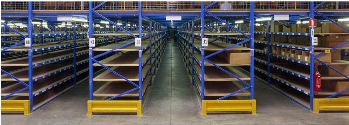
(a) Narrow-aisle racks
