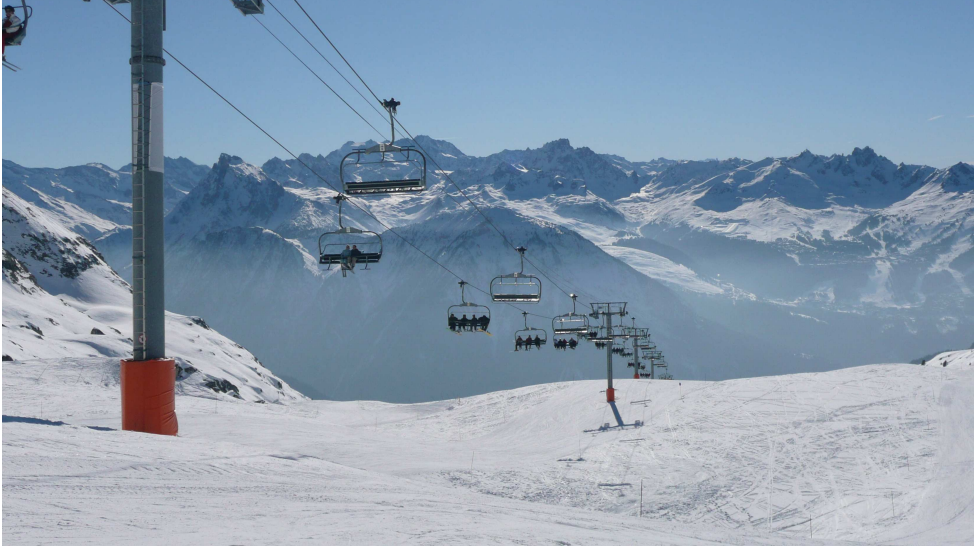
Figure 1.1: An example of a moving cable system.
