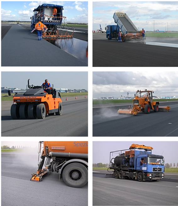
Figure 2.1: ASK installation proces
