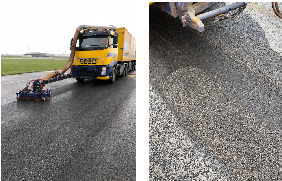
Figure 8.8: Waterjetting process and heterogeneity of TD surface
