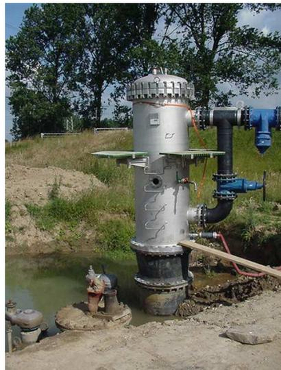
*Fig 5-8 Launce installation for pigs in a pressurised pipe*
