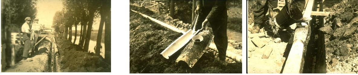
*Fig 7-1 Pre-1940 pipe laying with lead joint*
