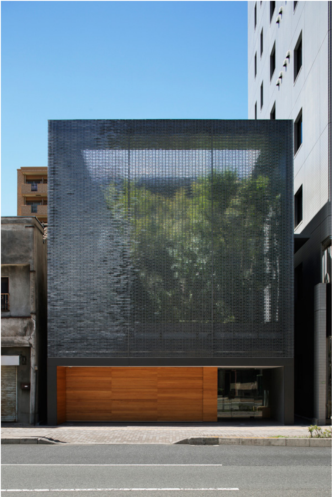
Figure 29: The glass brick facade in the Optical House. Source: HIROSHI NAKAMURA & NAP.
