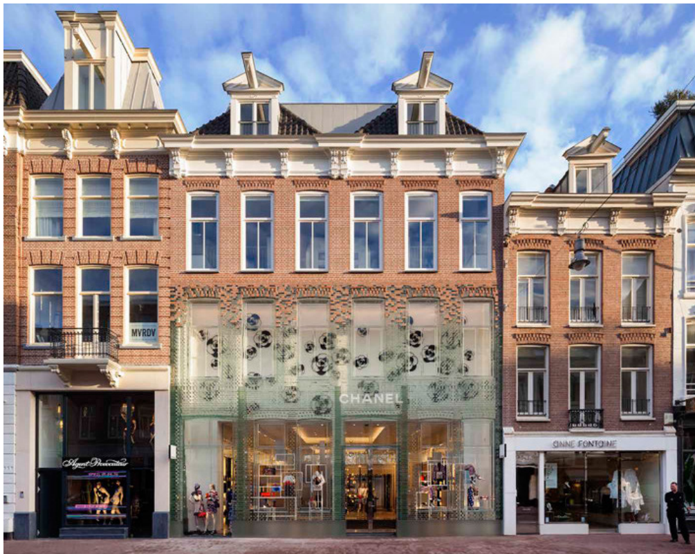
Figure 20: The Crystal Houses Facade in Amsterdam by MVRDV. Retrieved from (Oikonomopoulou, et al., 2018).
