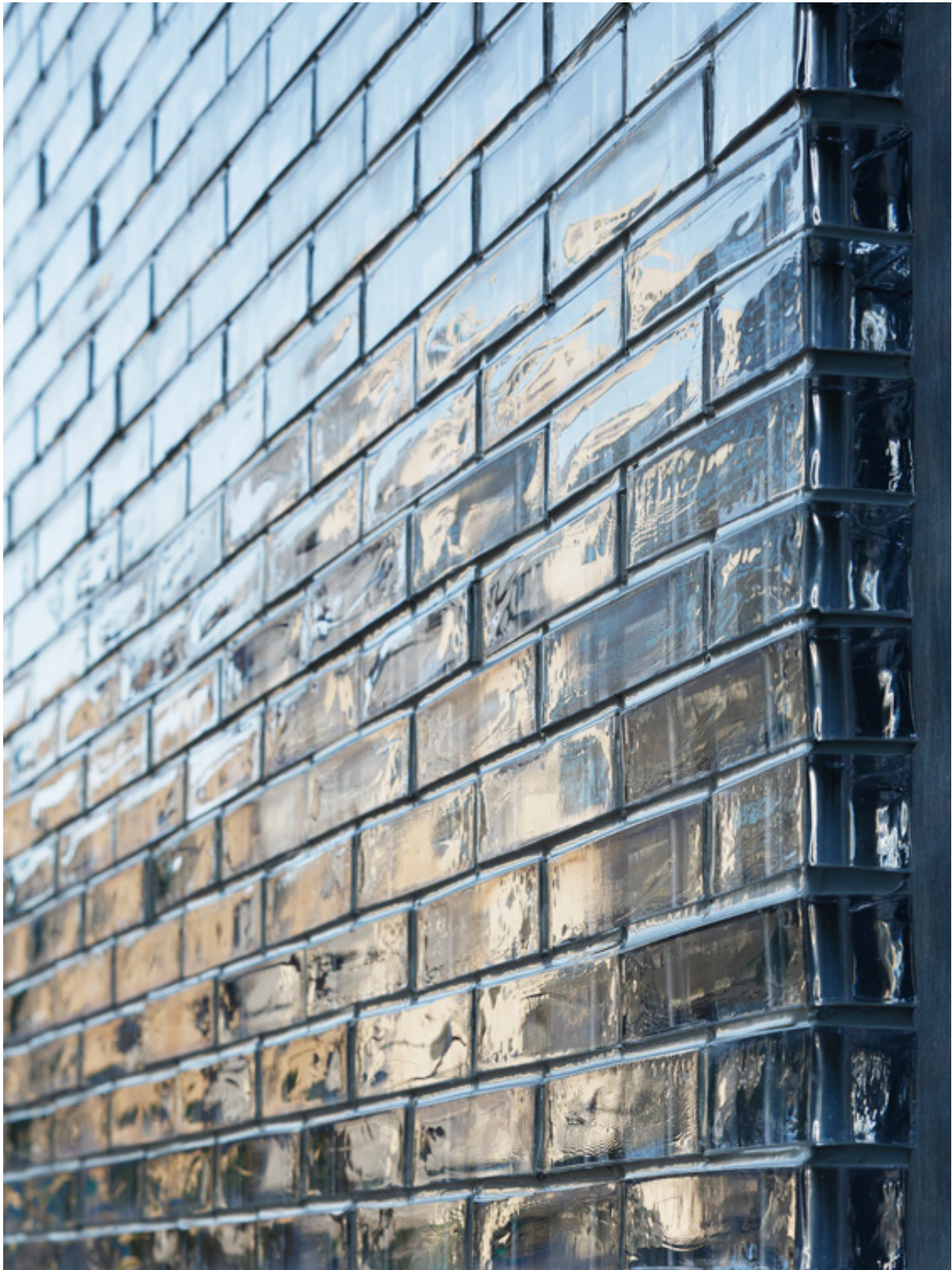
Figure 32: Supportive substructure in cast glass structures in the Optical House. Source: HIROSHI NAKAMURA & NAP.
