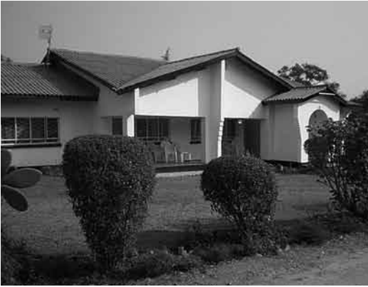
High-cost housing in Riverside, Kitwe.
