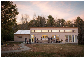
Fig.17: Images of Go_logic houses and planar element installation [20]
