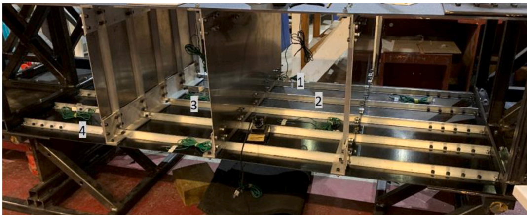
Fig. 13. Location of debonded stiffeners.
