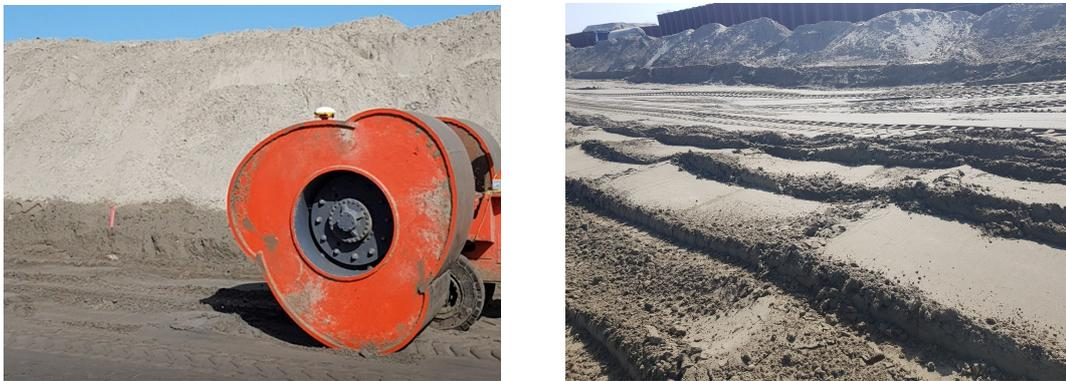
Figure 3.5: Heaving and loosening of the topsoil due to the motion of the roller
