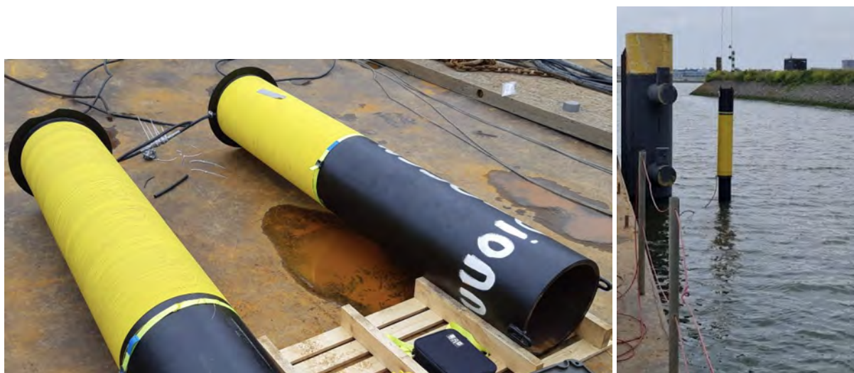
Figure 1 Left: two mantles of which only the right one is used. Right: picture of a mantle being installed on a pole.
