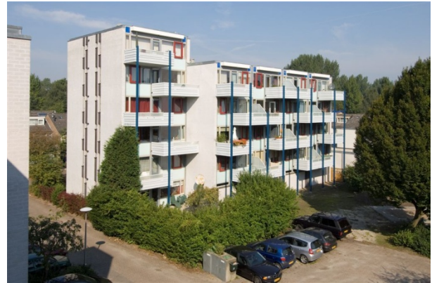
Figure 2-29: Acaciaplein, after renovation (Nationale Renovatie Prijs)
