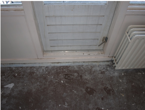
Figure 4-27: Door at the balcony (by author)
