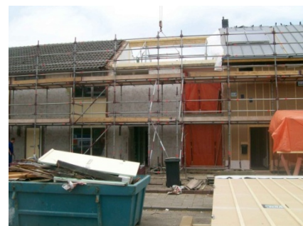
Figure 2-19: Kroeven 505 during refurbishment
