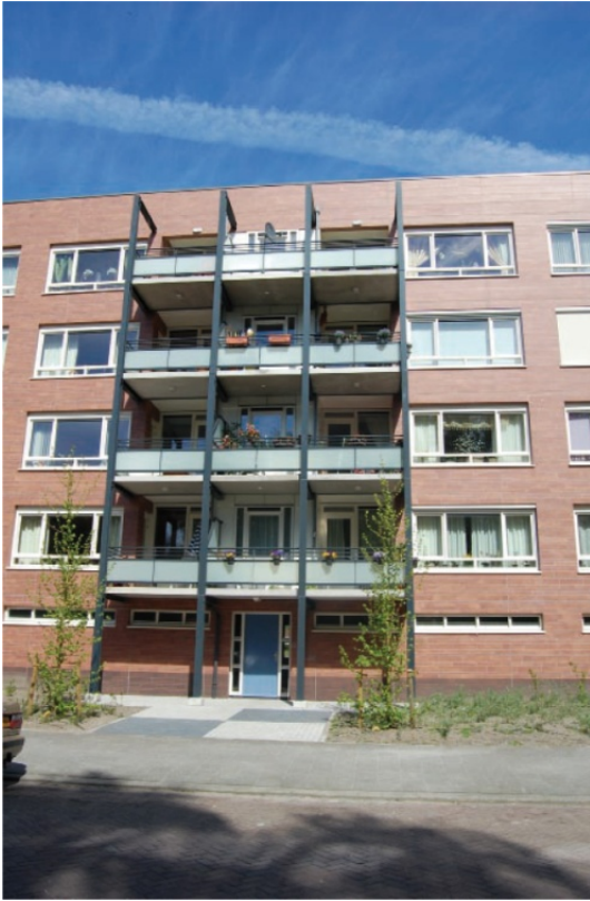
Figure 2-36: New situation Beatrixlaan, balcony construction (Van Bokhoven, 2009)
