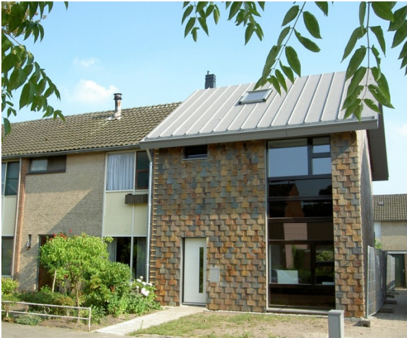
Figure 2-15: Kroeven Complex 505, before refurbishment (left) and after refurbishment (right) (DAT Architecten, 2007)
