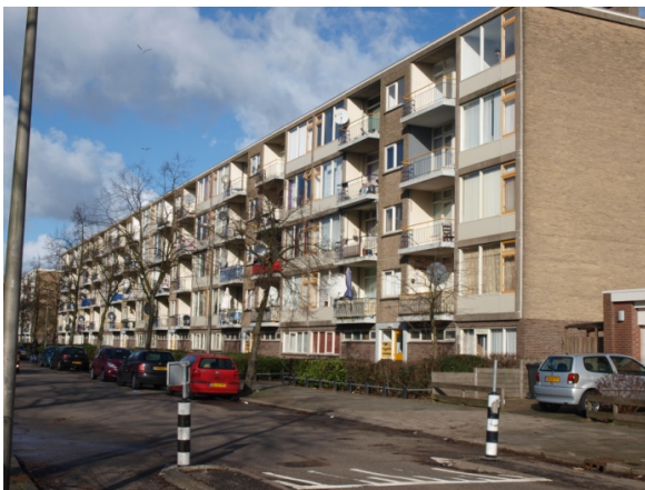
Figure 4-5: Front/west façade of the building (by author)
