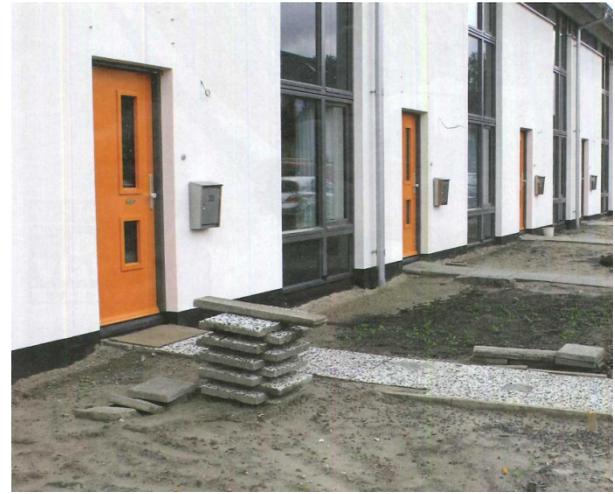
Figure 2-16: Kroeven complex 506 after refurbishment (Bol, 2010)
