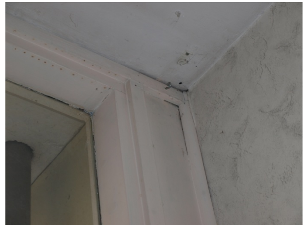
Figure 4-28: Top of the window frame in the living room (by author)
