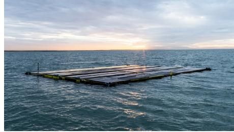
(b) Offshore floating PV system installed by Oceans of Energy in the North Sea [53]
