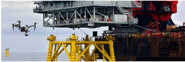
Fig. 3: Drones as an installation aid
