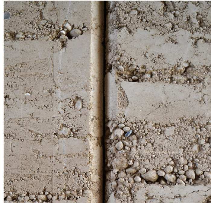
Limburg earth - rammed earth construction
