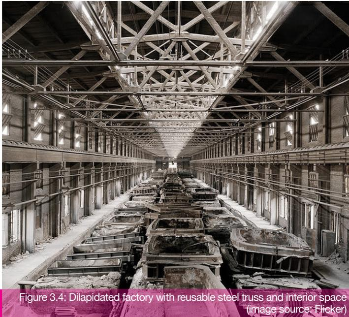
Figure 3.4: Dilapidated factory with reusable steel truss and interior space
