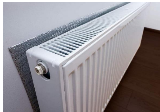
Figure 6.9: Transmission losses through the wall by a radiator (Duurzaam Bouwloket BV, n.d.)
