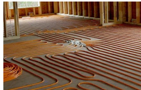
Figure 6.15: Floor heating (Watts, n.d.)
