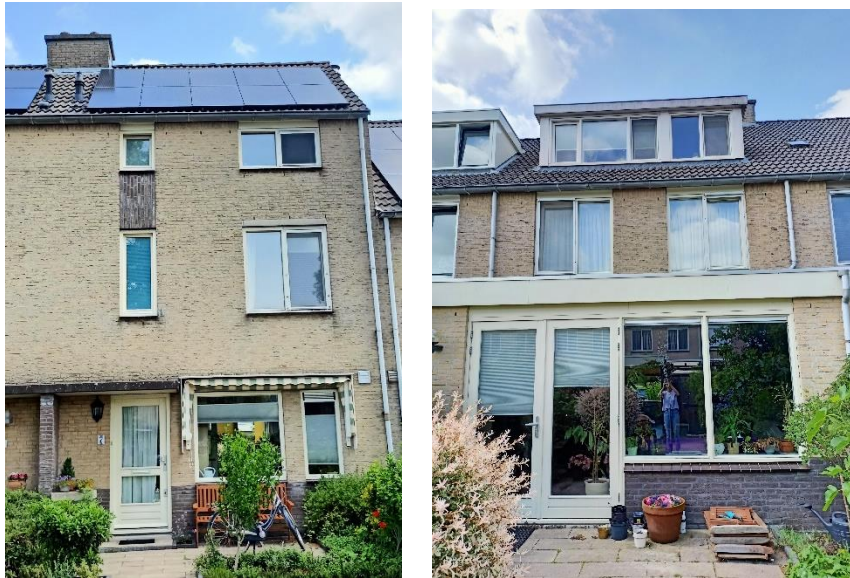
Figure 16.1: Case study building
