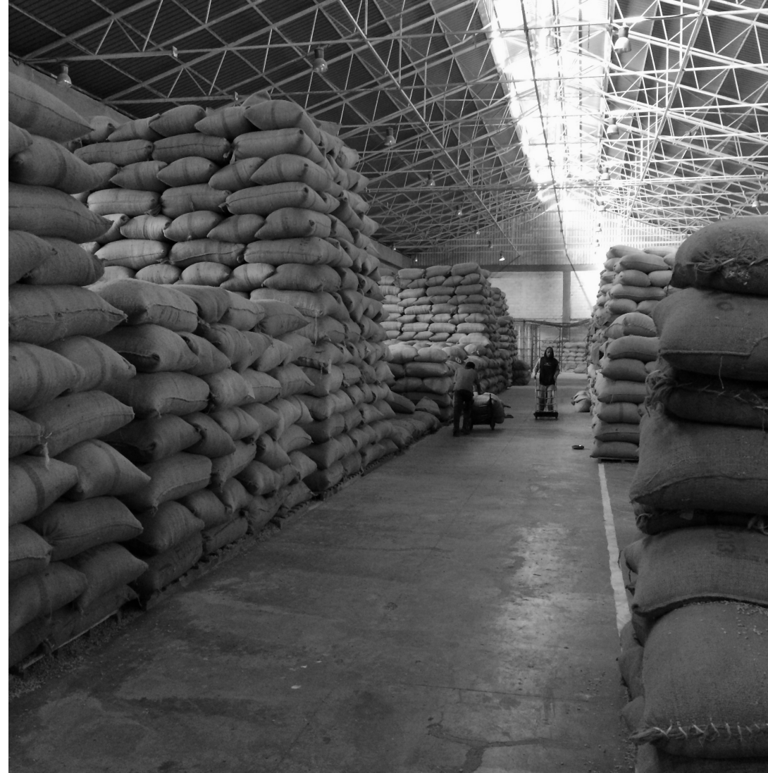
Central Warehouses for non-perishable produce , Nashik
