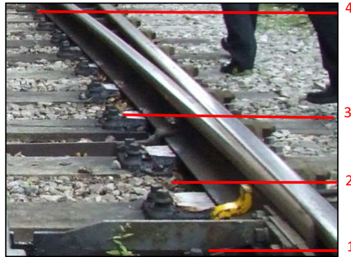
Figure 4.11: The positions of the four cases in the turnout: (1) before the turnout on a tangent track; (2) at the point where the wheel first makes contact with the switch blade; (3) on the switch blade; and (4) in the turnout when all transient phenomena have faded out.
