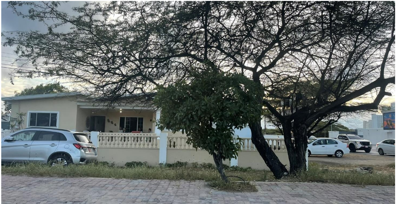
Figure 3. An Aruban veranda with a combination of a wall and a decorative balustrade, Aruba. Photograph by author, December 30, 2024.
