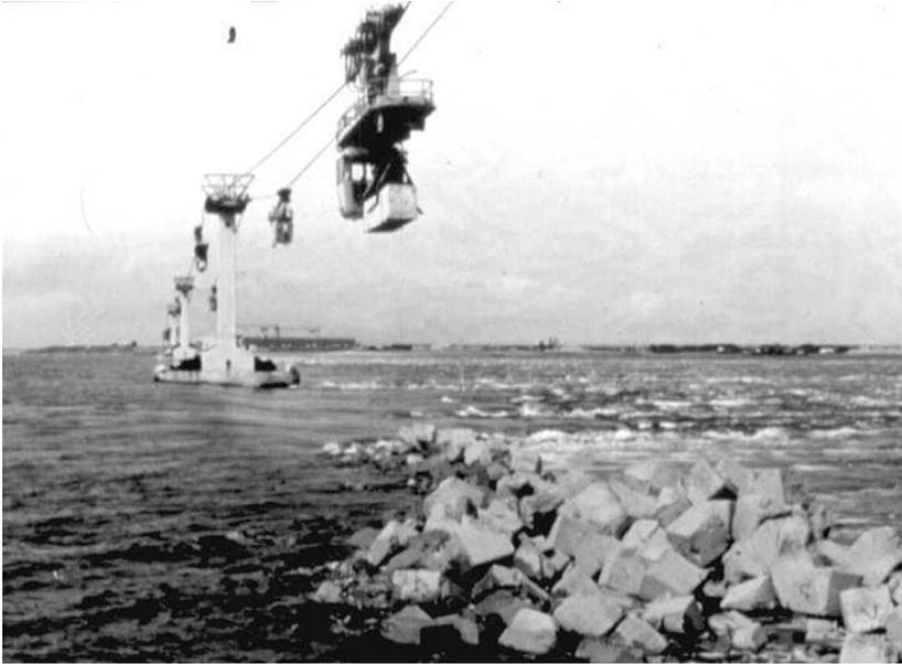
Figure 13-13 Closure with a cable way.
