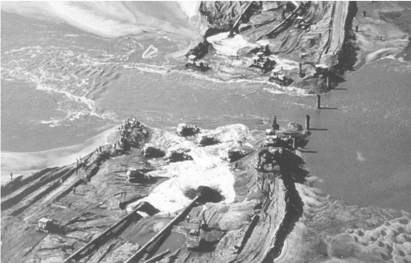
Figure 13-12 Final closure using sand only.
