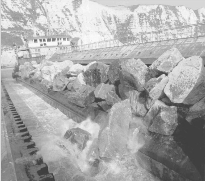
Figure A7-10 Side stone dumping vessel Cetus, dumping 1-3 t armourstone near a jetty (Royal Boskalis Westminster).
