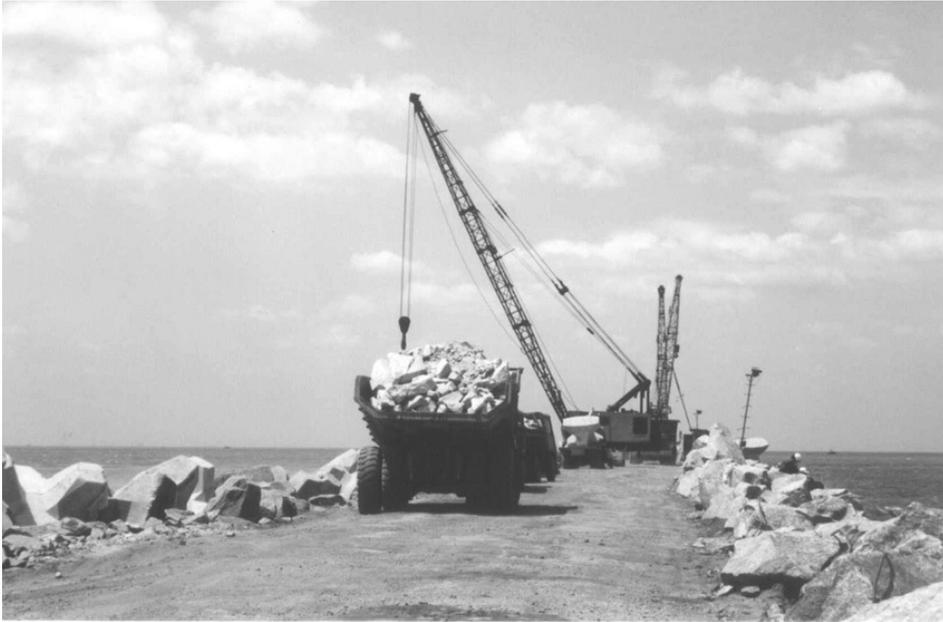
Figure 13-4 A breakwater under construction.
