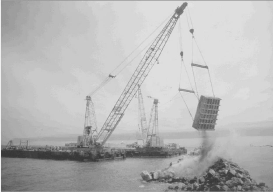
Figure A7-7 Placing armourstone from floating barge using a rock tray/skip.
