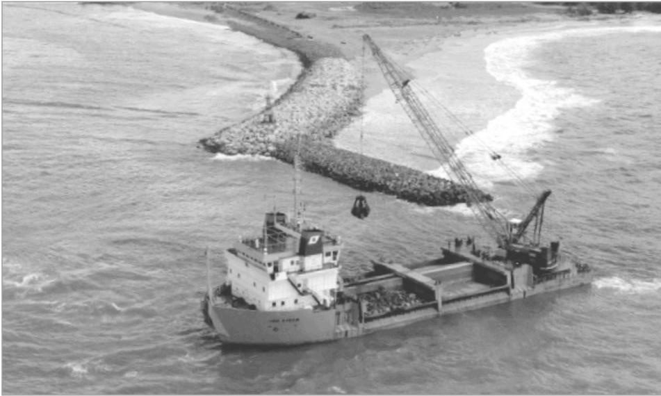
Figure A7-12 Crane mounted on the rock supply vessel Jan Steen (Van Oord).
