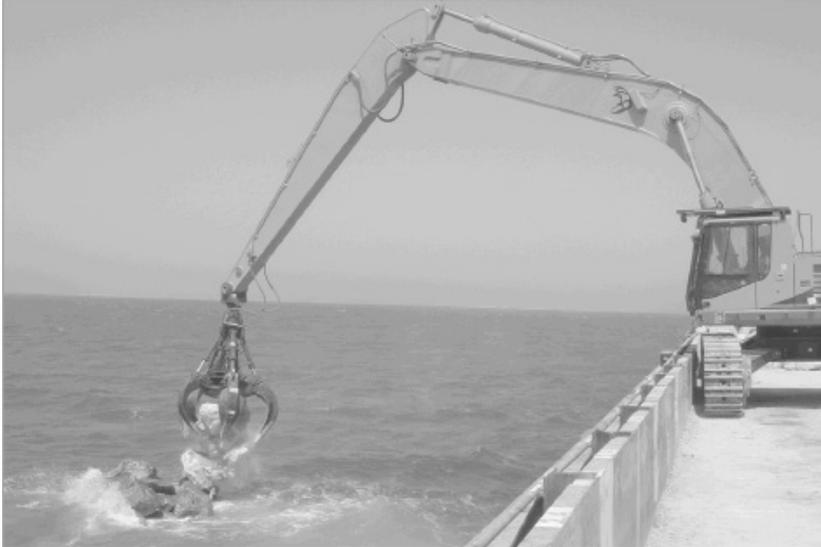
Figure A7-11 Placing armourstone with an excavator (Van Oord).
