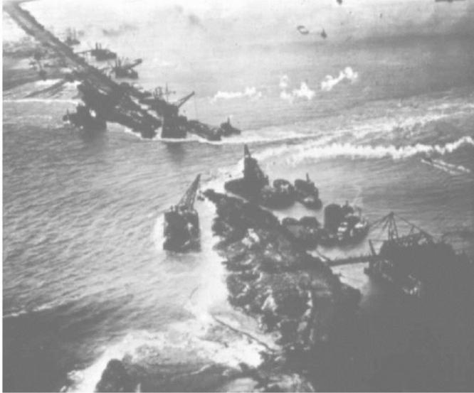
Figure 5-2 Flow through a closure gap.
