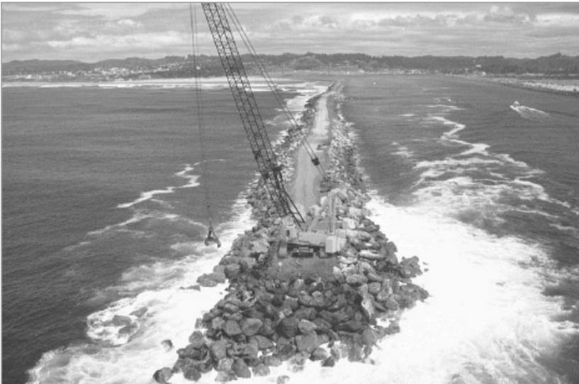
Figure A7-4 Crawler crane working on breakwater crest (courtesy Brien Wegner, USACE).
