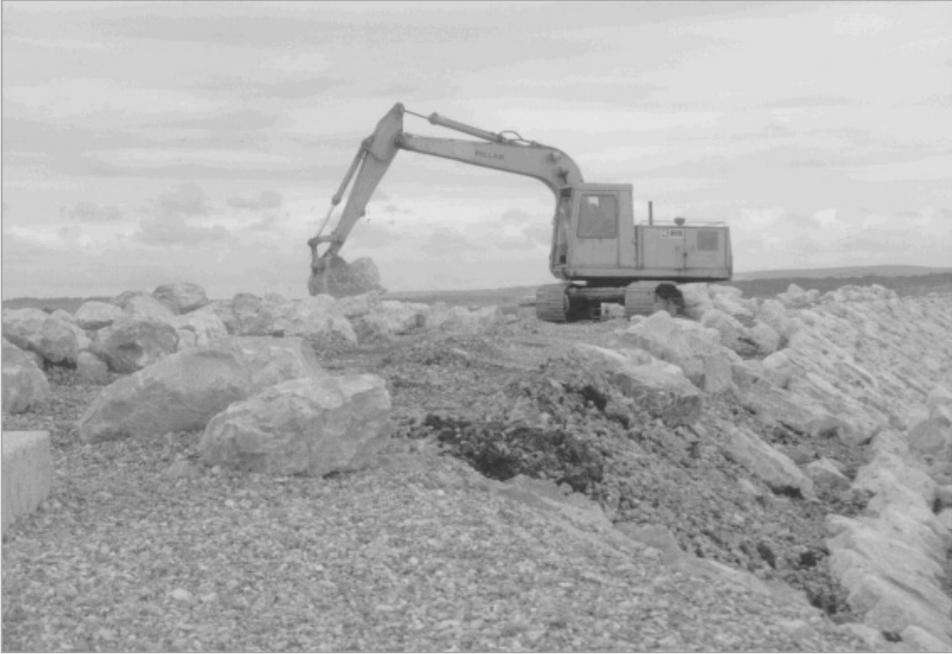
Figure A7-3 Excavator working on the crest (courtesy J.D. Simm).
