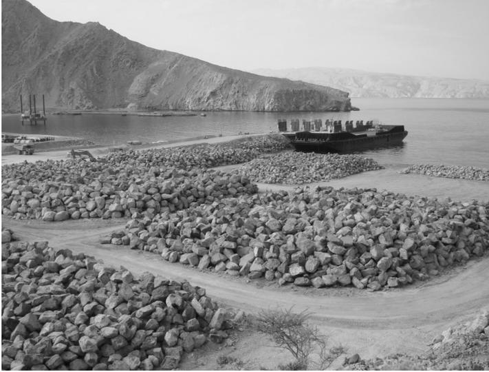
Figure 13-2 Stockpile area with wide gradings.
