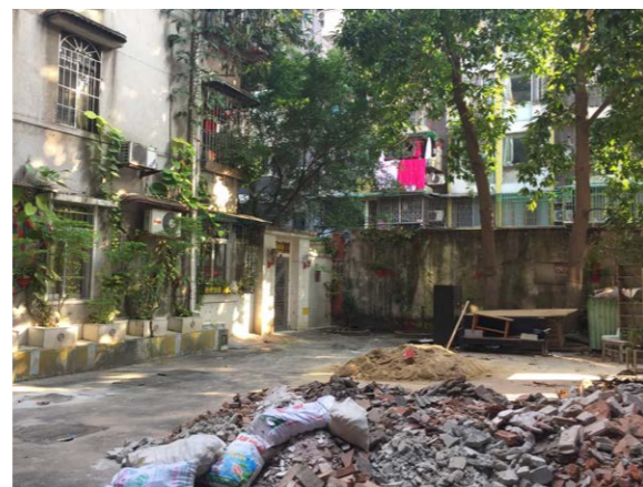
fig16. public space blocked with construction waste Source: author
