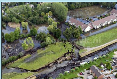
Figure 18: Regional flood defence breach at Wilnis, 2003 (Source: KoenSuyk photography)
