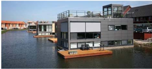
Figure 5.13: open tray caissons
