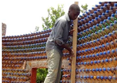
Figure 5.8: PET bottles as building material
