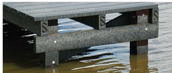
Figure 10.11: WPC submerged structure
