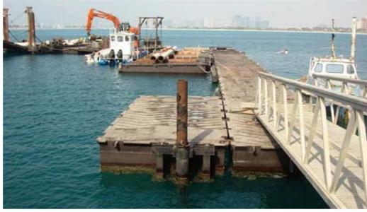
Figure 5.5: steel watertight caisson
