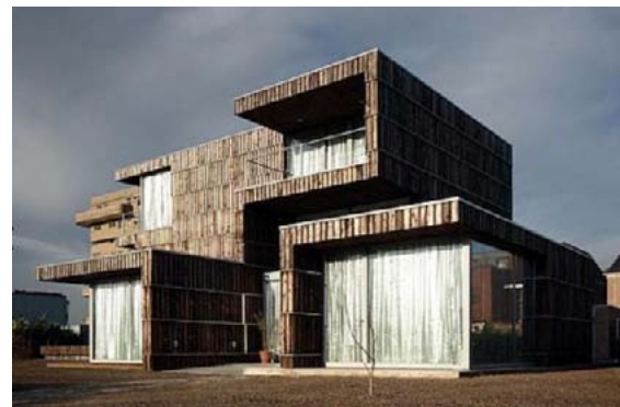
Fig. 2 Step 2: Experimentation Phase. Villa Welpeloo by 2012 Architects made of recycled textile, wood, flooring and insulation
