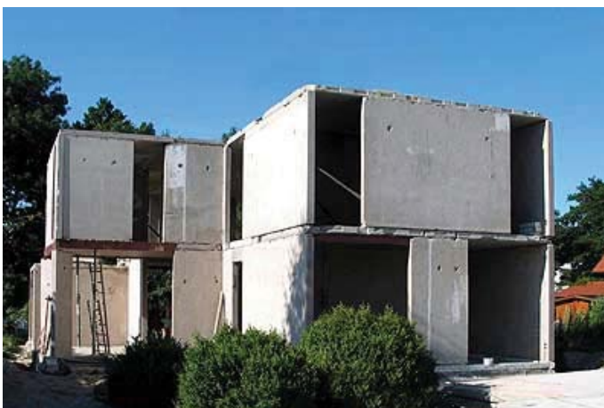
Fig. 83. recycled house in progress. source: conclus architekturbuero
