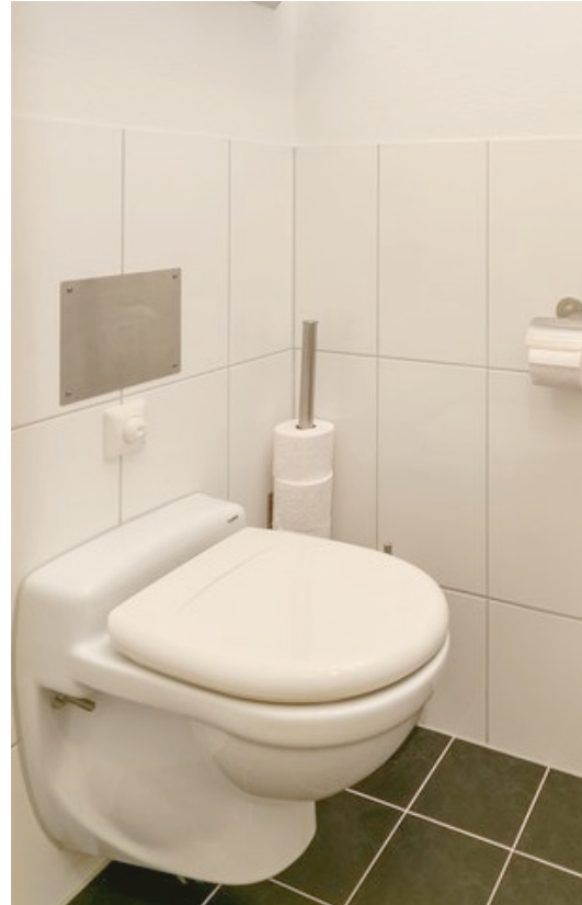
J. Vacuum toilet in the 'Casa Vita' building in Deventer (photo by Helder Makelaars, 2019)
