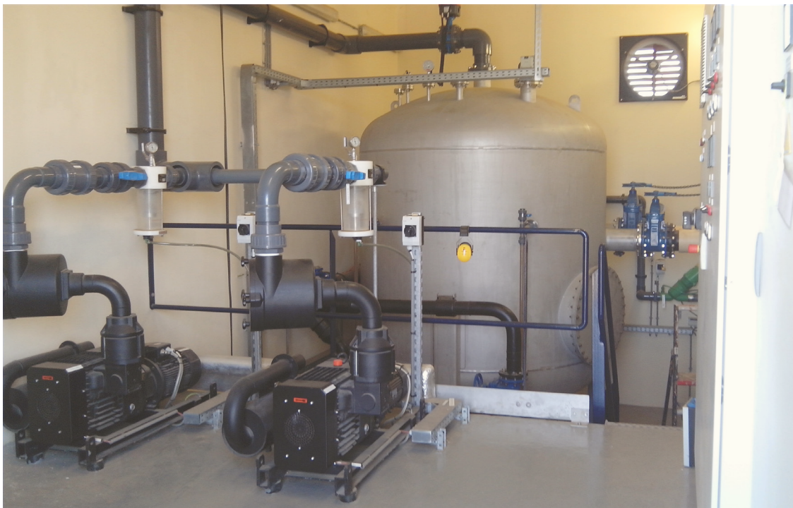
K. Pumping station of a vacuum sewer (photo by Dieks)
