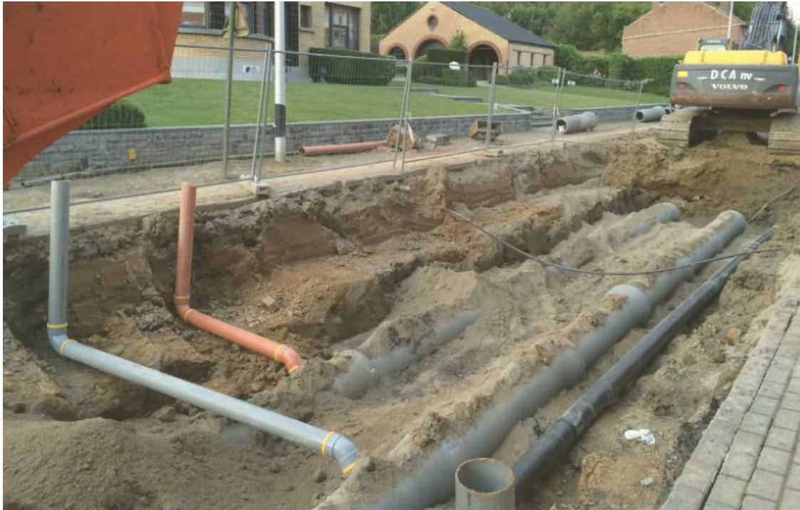
L. Conventional (separated) gravitational sewer (photo by ACA VZW)
