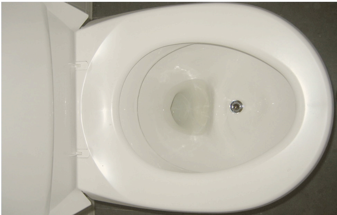
H. Urine diverting toilet in the Waterboard building in Meppel (photo by E. v. Münch, 2006)
