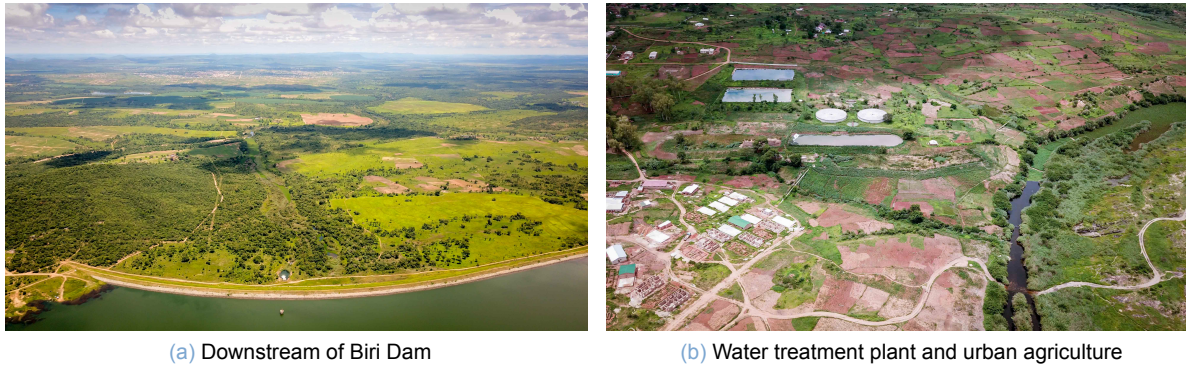
Figure 43: Downstream of Biri Dam from the sky
