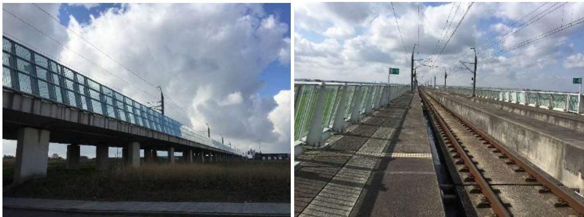
Figure 62: Two pictures of viaduct Bleiswijk, taken by the author during a site visit in March 2016.
