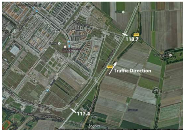
Figure 65: Aerial view of the damages near Zoetermeer (Google Maps)
