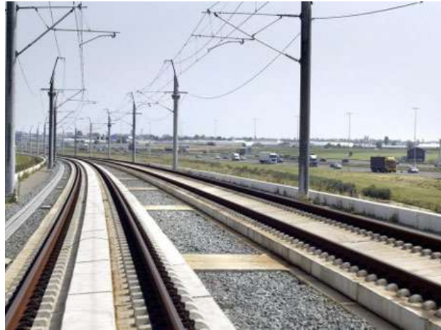
Figure 63: Rheda 2000 superstructure at a curve in the HSL-South. Source: http://www.rgprojecten.nl/images/projecten/rheda2000/HSL-002.jpg
