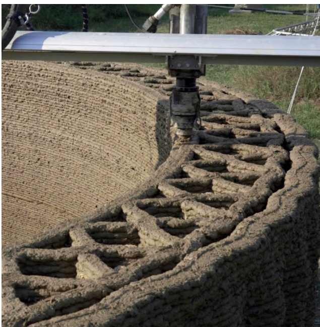
Figure 14. A Wasp 3D printer at work: Semper reinvented (Wasp, 2018).
