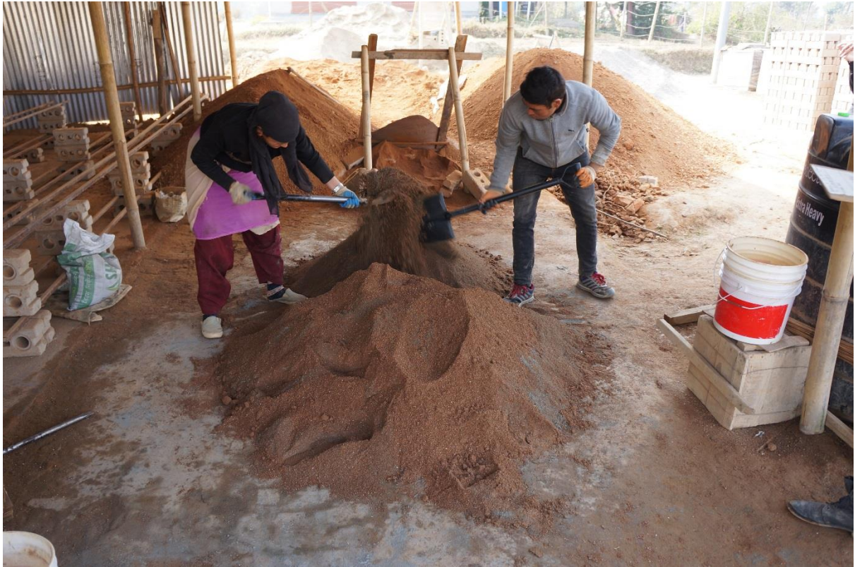
Figure 3: Nepali workers making the drymix for CSEB
