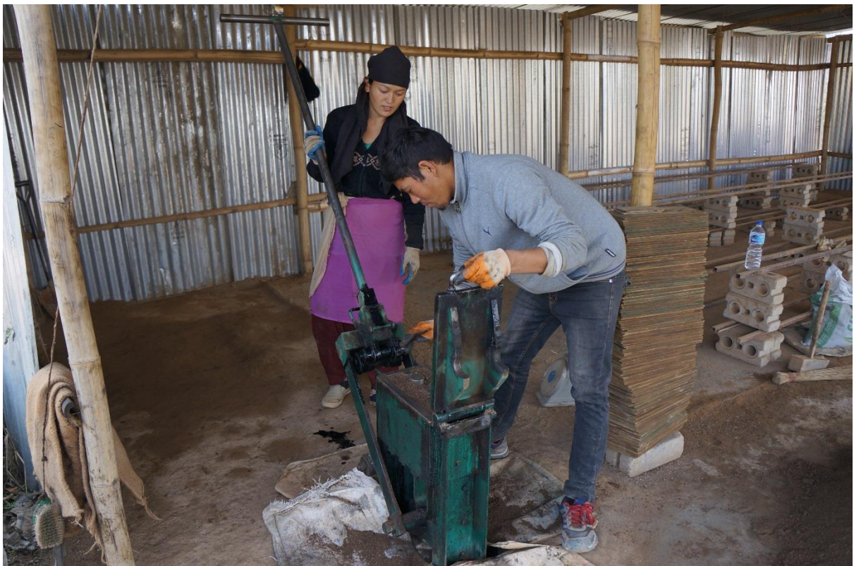
Figure 4: Nepali workers putting the mixture in the CSEB press
