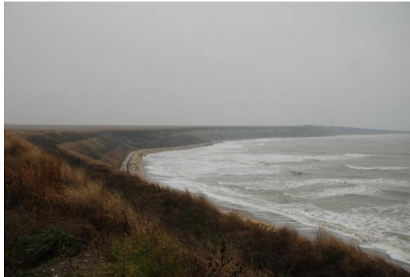
Fig. 3.38 Cliff protection at south of Tuzla Cape (southern Romanian coast) (original)
