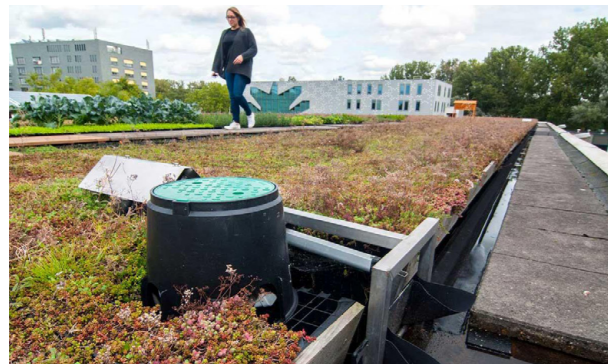
Figure 107. Example of polder roof in Zuidas, Amsterdam. Source: dakdokters.nl
