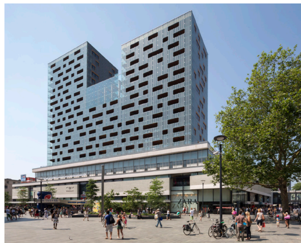
Figure 58. De Karel Doorman building in Rotterdam by Ibelings van Tilburg architecten. Addition of new layers over existing building. Source: www.archdaily.com
