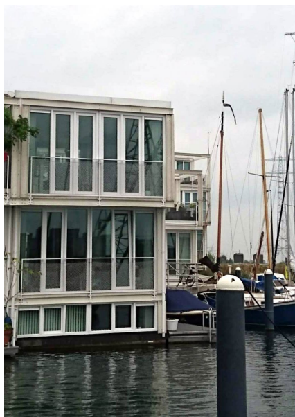
Figure 11. Waterwoningen Steigereiland by Marlies Rohmer, own picture
