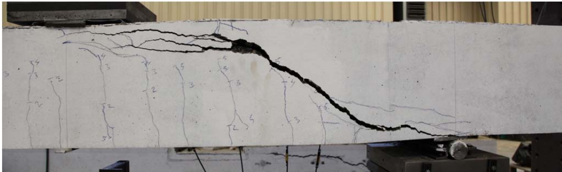
Fig. 5.17.2. Crack pattern after failure south side
