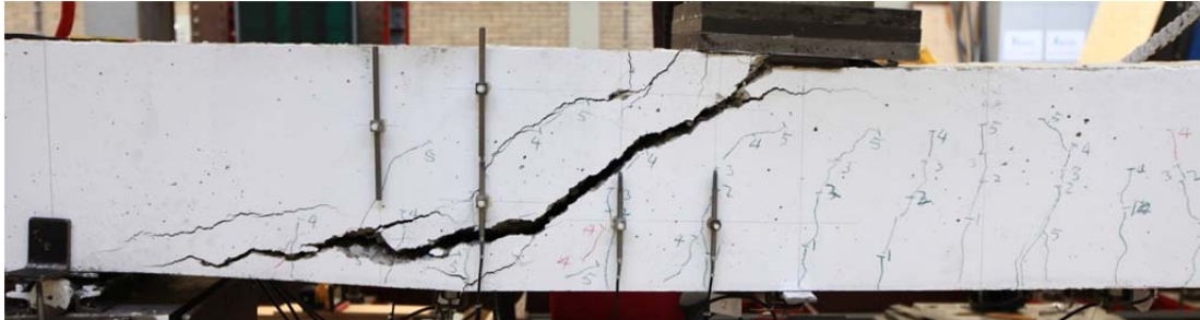
Fig. 5.55.1. Crack pattern after failure north side
