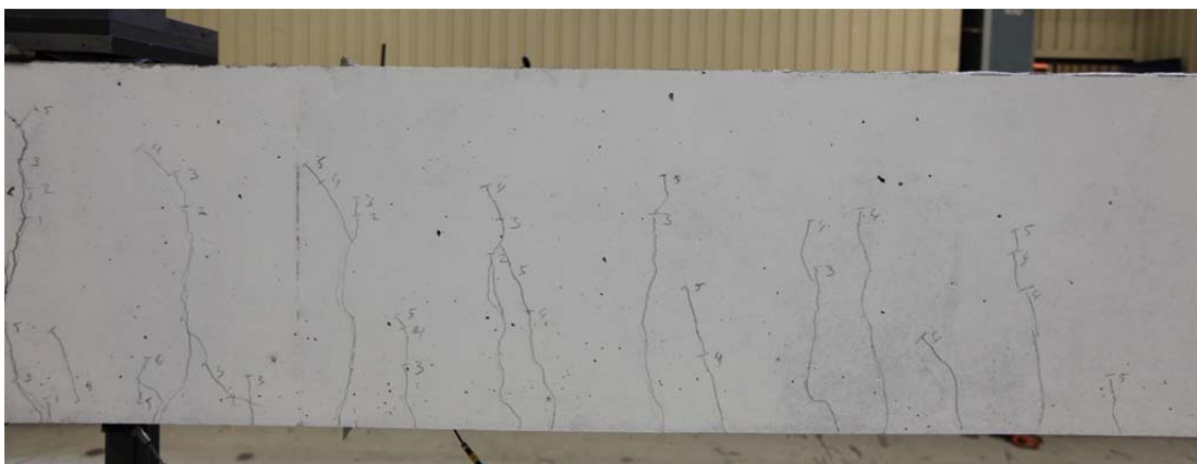
Fig. 5.40.2. Crack pattern after failure south side
