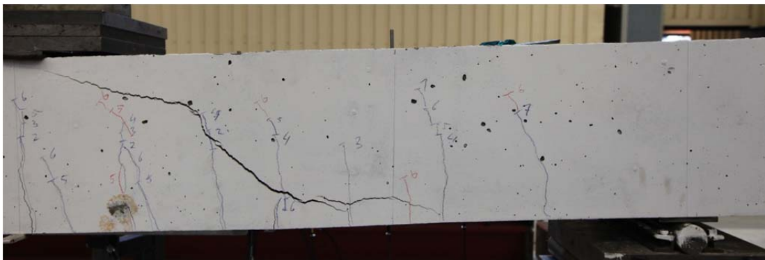
Fig. 5.11.2. Crack pattern after failure south side
