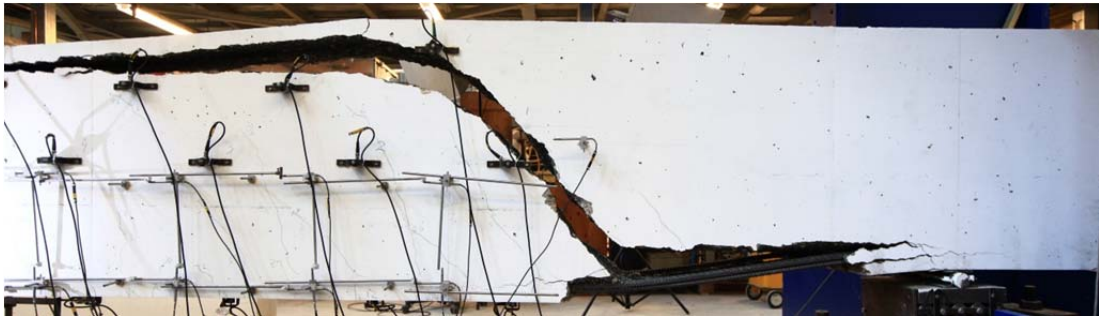
Fig. 5.104.2. Crack pattern after failure and LVDT layout at west side of beam
