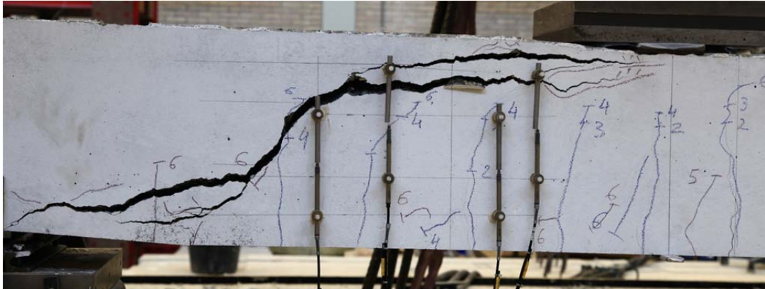
Fig. 5.21.1. Crack pattern after failure north side
