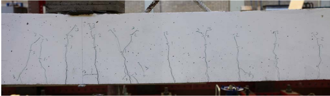
Fig. 5.62.1. Crack pattern after failure north side
