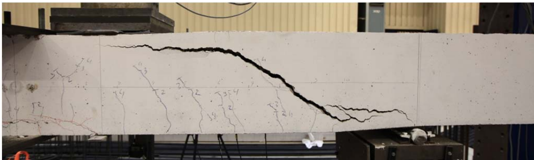
Fig. 5.56.2. Crack pattern after failure south side
