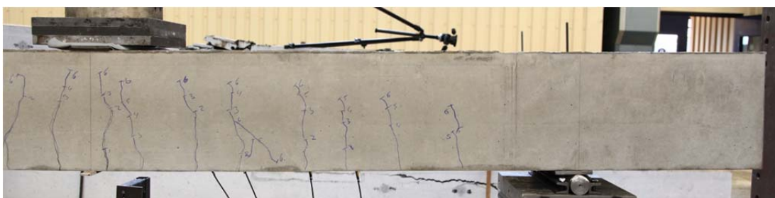
Fig. 5.12.2. Crack pattern after failure south side
