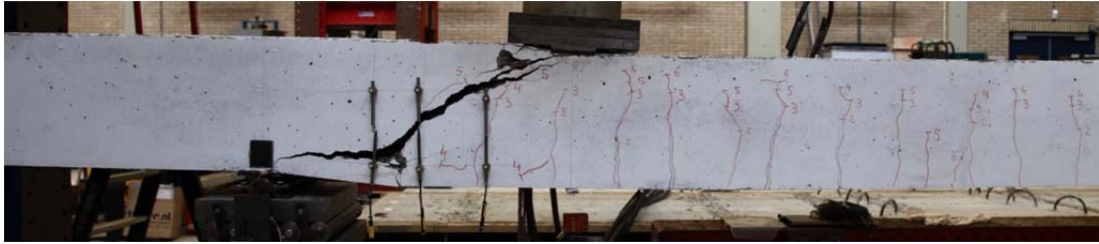
Fig. 5.33.1. Crack pattern after failure north side
