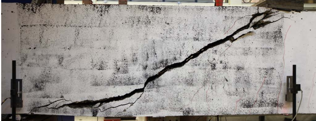
Fig. 5.103.1. Crack pattern after failure at north side of beam
