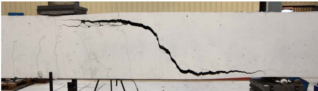
Fig. 5.49.2. Crack pattern after failure south side
