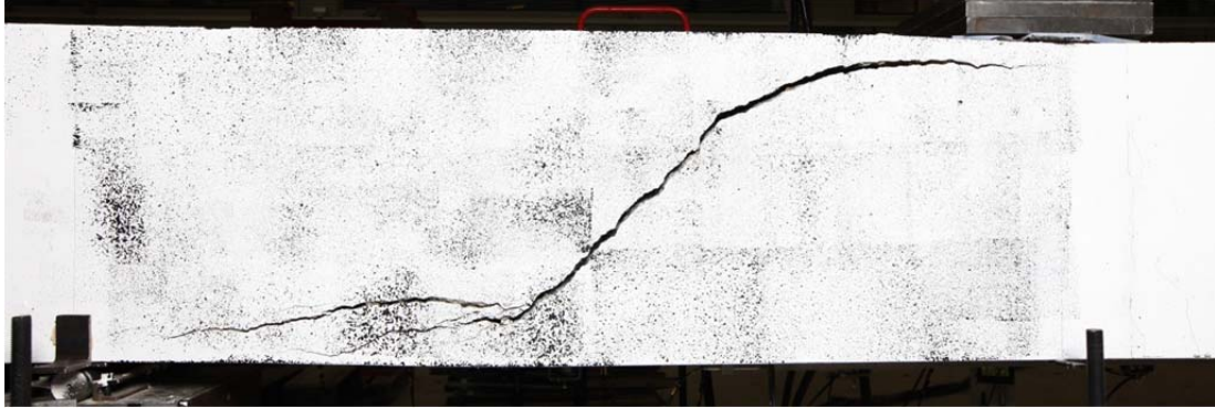
Fig. 5.96.1. Crack pattern after failure north side
