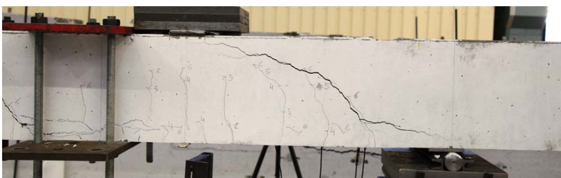
Fig. 5.7.2. Crack pattern after failure south side
