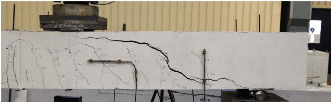
Fig. 5.3.2. Crack pattern after failure south side
