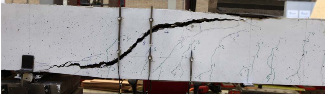
Fig. 5.59.1. Crack pattern after failure north side
