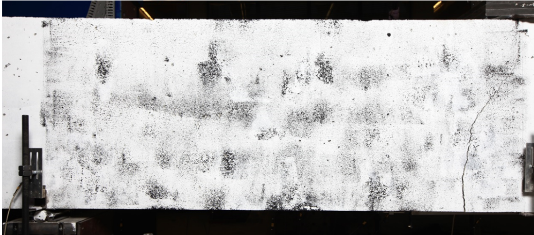
Fig. 5.83.1. Crack pattern after failure north side
