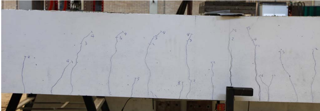
Fig. 5.47.1. Crack pattern after failure north side
