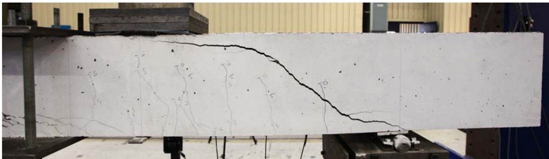
Fig. 5.9.2. Crack pattern after failure south side
