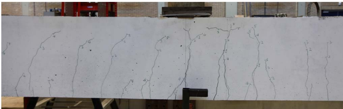
Fig. 5.41.1. Crack pattern after failure north side
