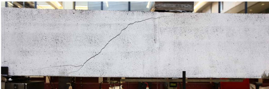
Fig. 5.77.1. Crack pattern after failure front side
