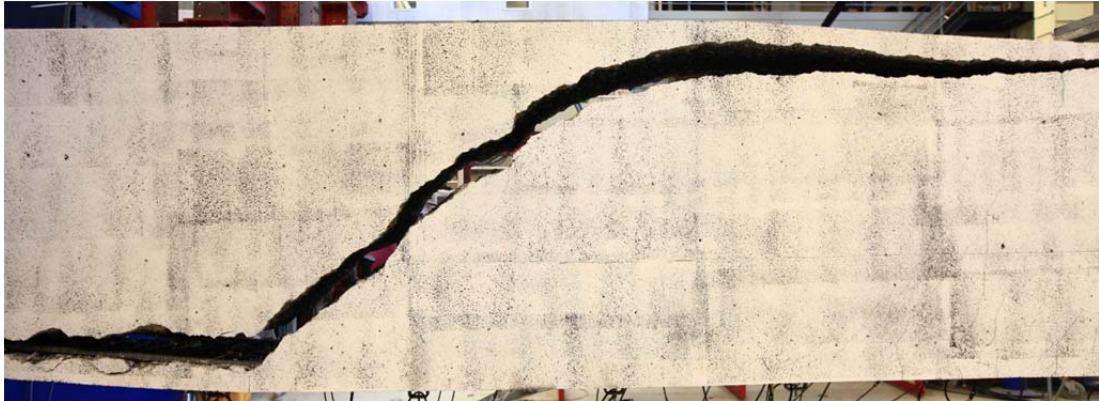
Fig. 5.105.1. Crack pattern after failure at east side of beam
