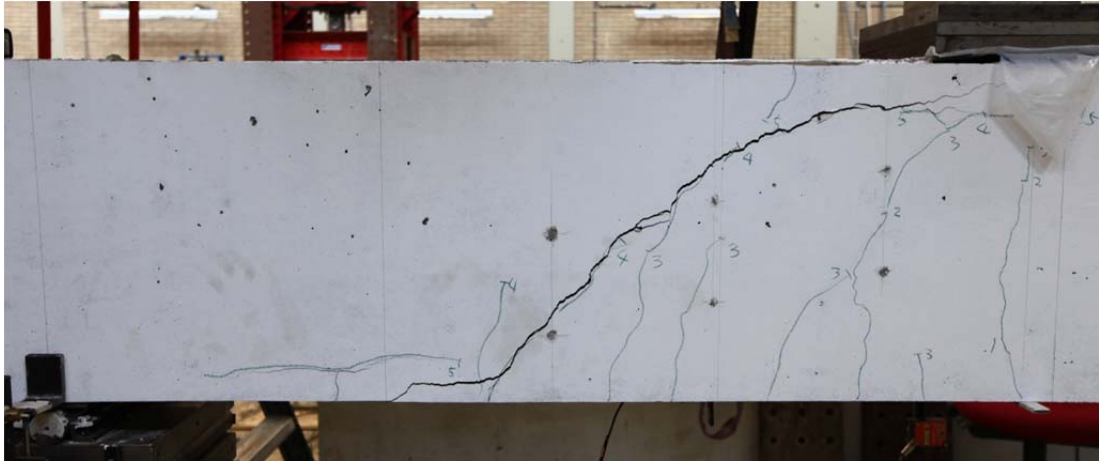
Fig. 5.46.1. Crack pattern after failure north side
