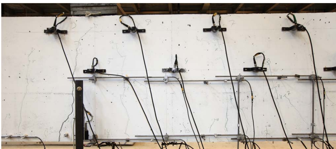
Fig. 5.92.2. Crack pattern after failure west side
