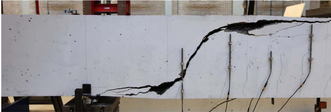
Fig. 5.53.1. Crack pattern after failure north side
