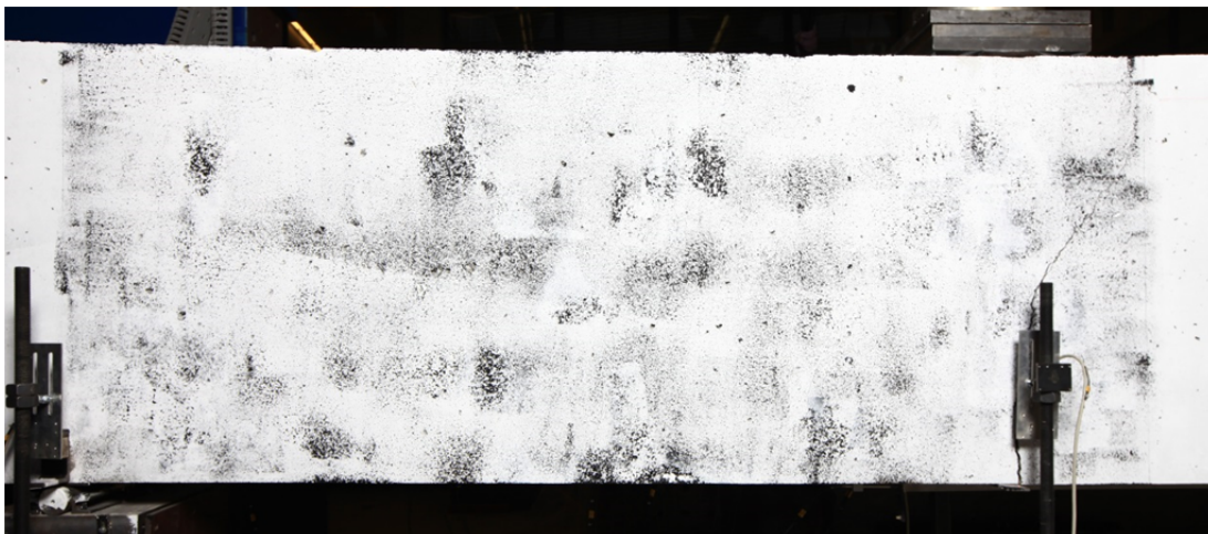
Fig. 5.84.1. Crack pattern after failure north side
