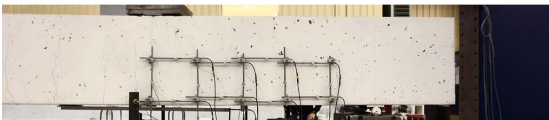
Fig. 5.80.2. Crack pattern after failure back side
