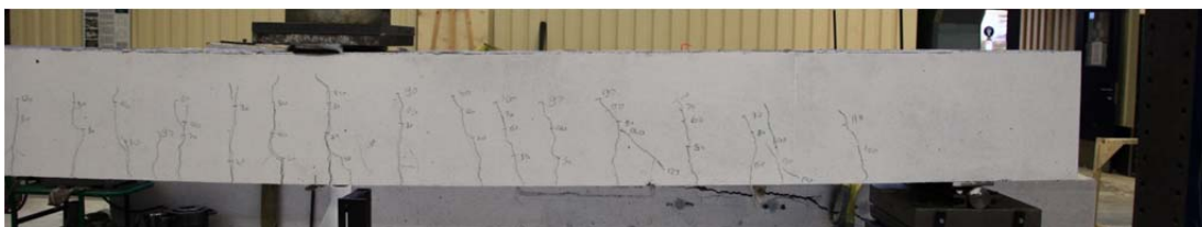
Fig. 5.1.2. Crack pattern after failure south side
