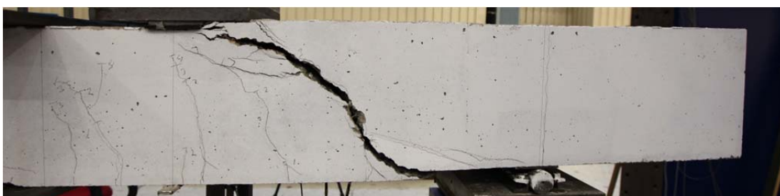
Fig. 5.65.2. Crack pattern after failure south side
