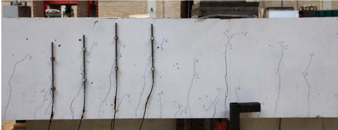
Fig. 5.43.1. Crack pattern after failure north side
