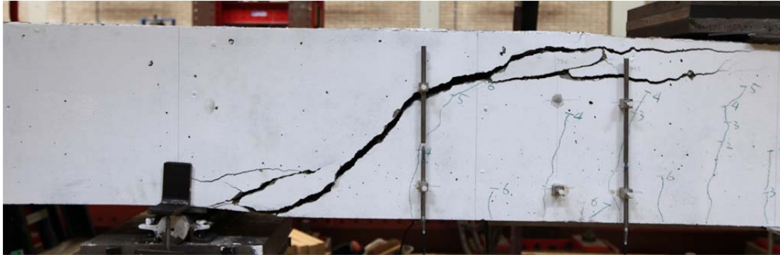
Fig. 5.8.1. Crack pattern after failure north side
