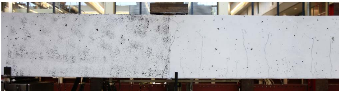
Fig. 5.80.1. Crack pattern after failure front side
