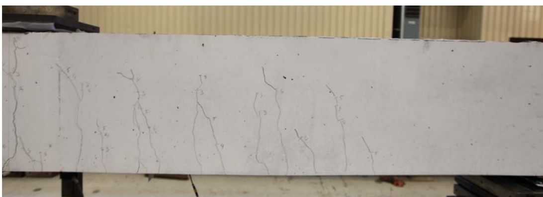
Fig. 5.41.2. Crack pattern after failure south side
