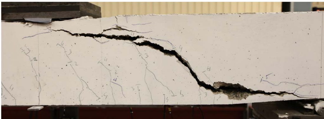
Fig. 5.59.2. Crack pattern after failure south side
