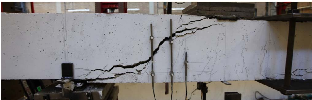
Fig. 5.65.1. Crack pattern after failure north side
