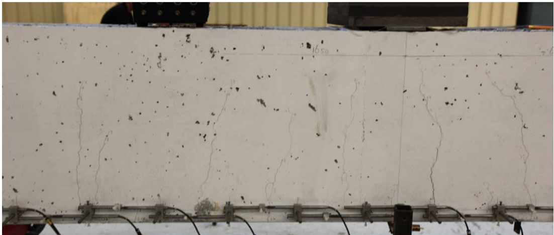
Fig. 5.82.2. Crack pattern after failure south side
