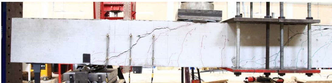
Fig. 5.16.1. Crack pattern after failure north side
