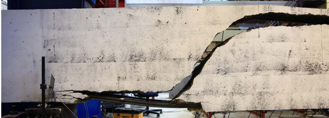
Fig. 5.104.1. Crack pattern after failure at east side of beam
