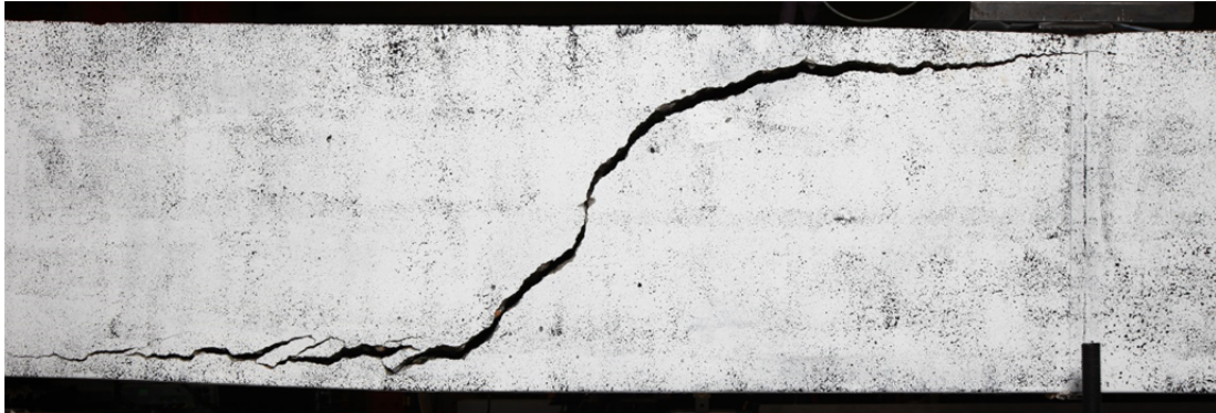
Fig. 5.98.1. Crack pattern after failure north side
