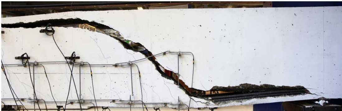
Fig. 5.105.2. Crack pattern after failure and LVDT layout at west side of beam
