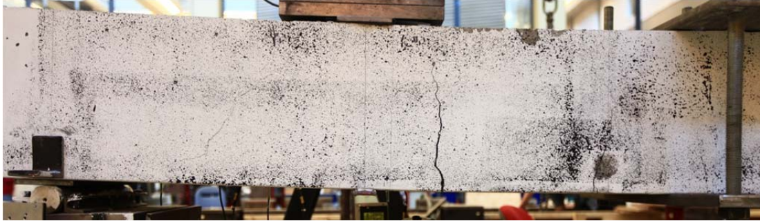
Fig. 5.74.1. Crack pattern after failure front side
