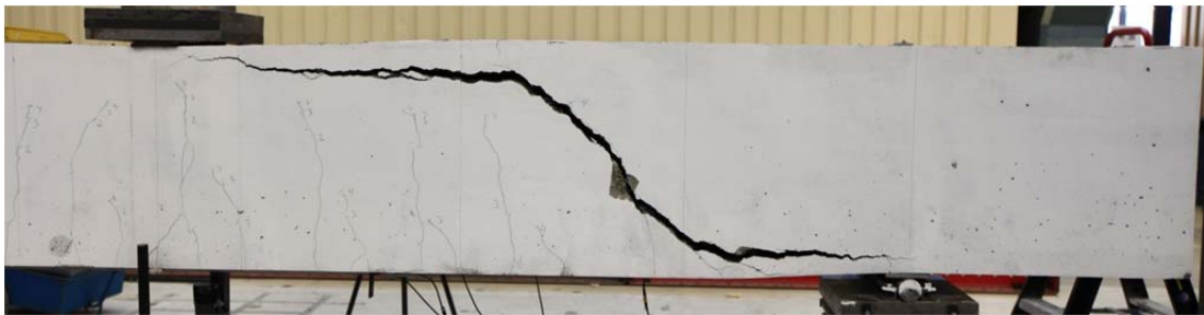
Fig. 5.53.2. Crack pattern after failure south side
