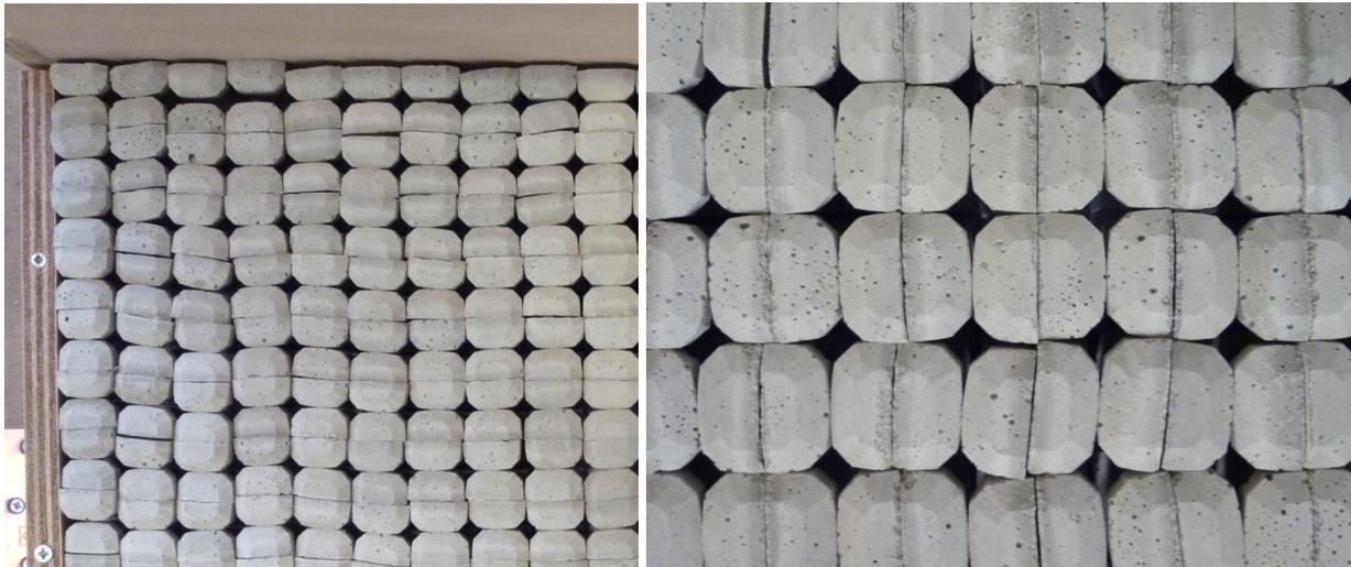
**Figure 2-6: Hillblock revetment with standard placement (left) and rotated placement (right)**
