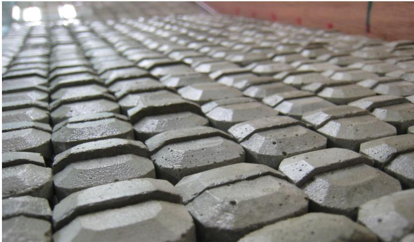
Figure 4-12: Hillblock revetment with modified placement pattern
