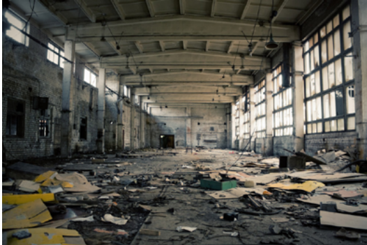
Fig. 5-2-3: Abandoned Industrial Heritages Source: http://img.taopic.com/uploads/allimg/121220/235035-1212200553432.jpg
