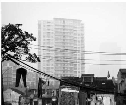
Shanghai Shikumen demolition Project (2004)
