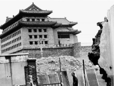
Demolition for creating 'available land' for new development Source: http://finance.people.com.cn/n/2012/0827/c1004-18837374.html
