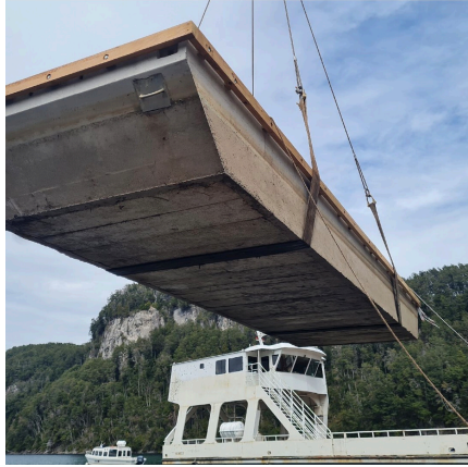
Figure 8.8: Installation of a floating breakwater (left) [41]. Concrete floating breakwater (right) [42]
