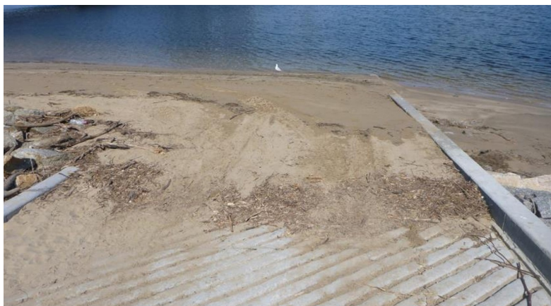
Figure 8.17: Boat ramp affected by sedimentation [51].
