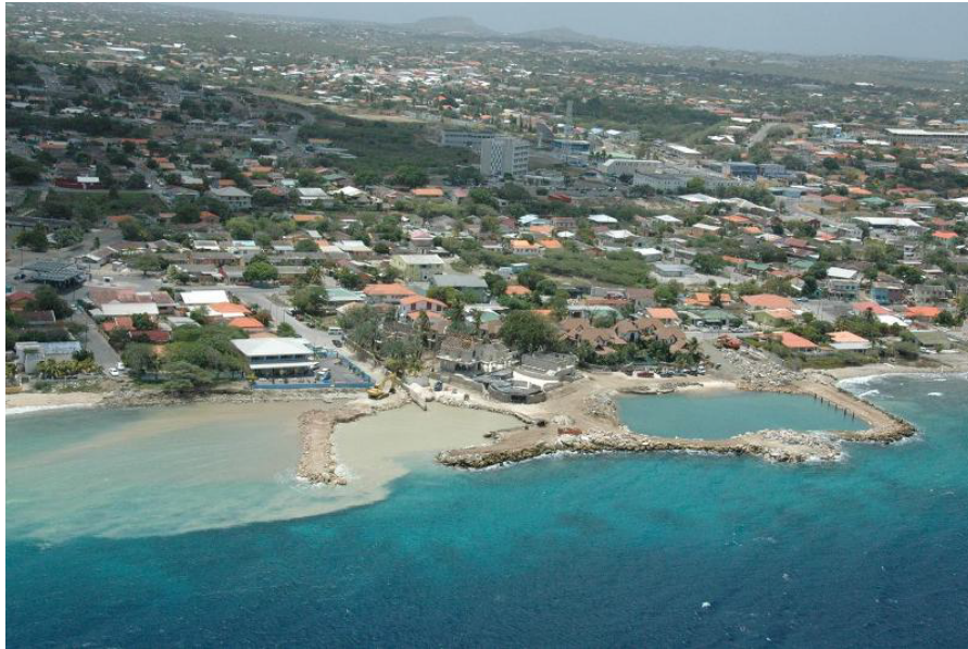
Figure 3.17: Photo taken in 2008, showing the effects of the construction activities at Baoase, source: ProMonumento
