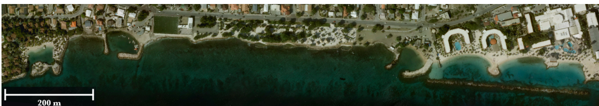
Figure 3.8: Aerial orthophotograph of the southwest coast from Baoase to Mambo beach in 2024, courtesy of CARMABI
