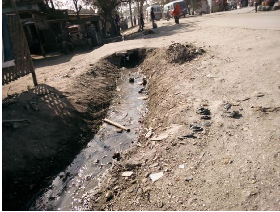
Figure 4.5: Example of a drainage ditch recorded by Ramani Huria . Photo by Ivan Gayton. https://wiki.openstreetmap.org/wiki/File:Drain_ditch_open.jpgfilehistory
