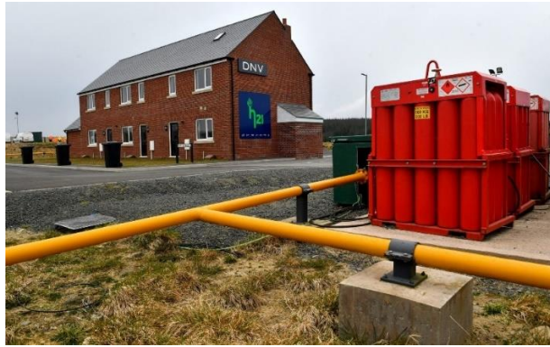
Figure 9. Hydrogen cylinders of H21 project by DNVGL. Retrieved from https://www.telegraph.co.uk/business/2021/05/03/hydrogen-heating-homes-pipeline/ accessed 29 March 2023
