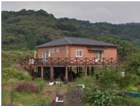
Stilt house in high flood risk area
