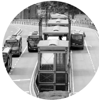
Advanced bus / trolley bus stops and stations
