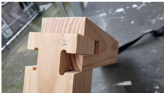
Figure 85 T joint Assembly
