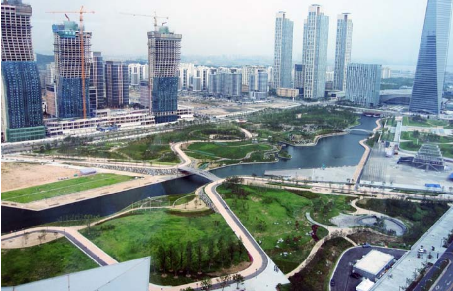
Figure 1. Songdo City in South Korea under construction, an airport-centric city to be completed in 2015. (Gale international and tk/pr public relations)
