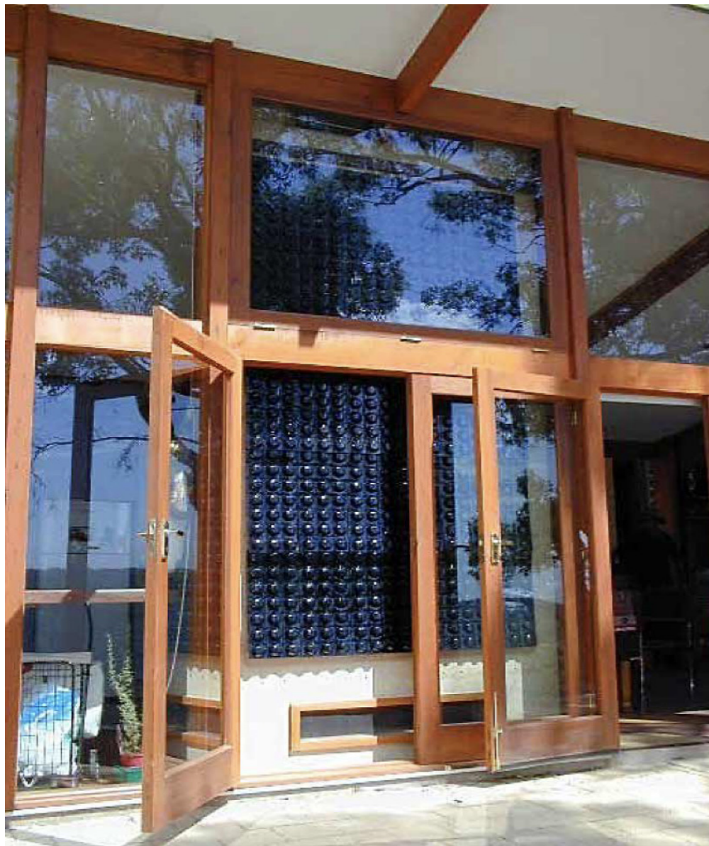
Figure 1.23 PCM modules on a thermal mass wall.. Reprinted from Energyarchitecture, n.d.. Retrieved from http://www.energyarchitecture.com.au/projects/norton-summit-ecological-footprint/
