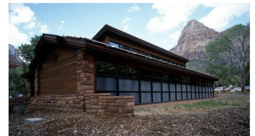
Figure 1.12 South facing Trombe wall Zion Visitor Centre. Reprinted from Green Building Brain, by R. Williamson, n.d.. Retrieved from https://greenbuildingbrain.org/buildings/zion_visitor_center
