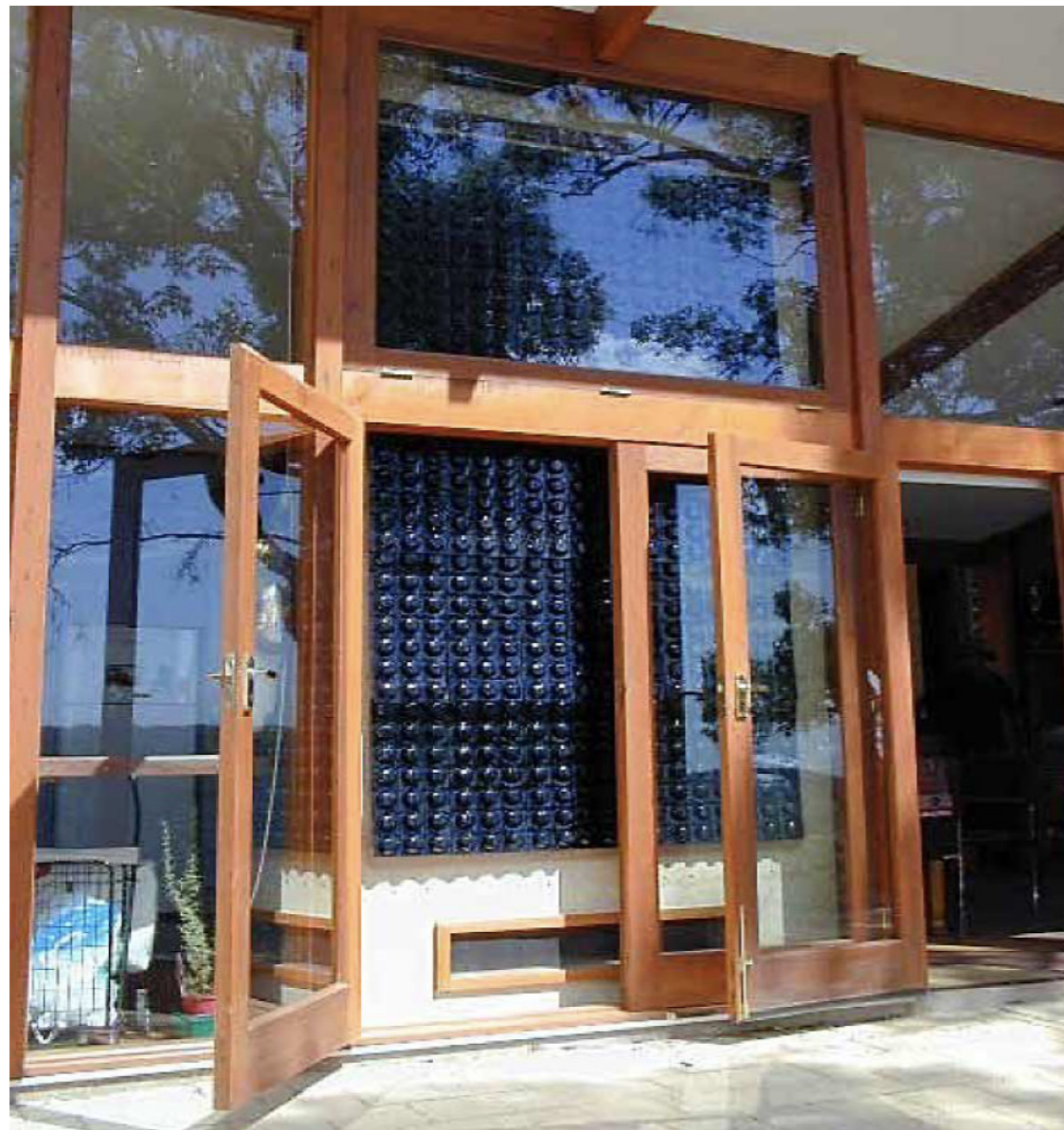
Figure 1.6 PCM modules on a thermal mass wall. Reprinted from Energyarchitecture, n.d.. Retrieved from http://www.energyarchitecture.com.au/projects/norton-summit-ecological-footprint/
