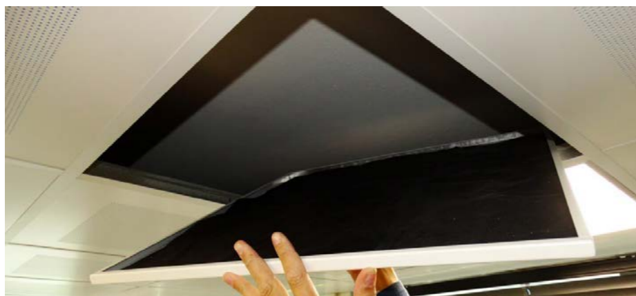
Figure 1.18 PCM ceiling system from Global-e-systems for both heating and cooling the space. Reprinted from Global-e-systems, by GES, n.d.. Retrieved from https://www.global-e-systems.com/en/products/thermavar-pcm-climate-ceiling/
