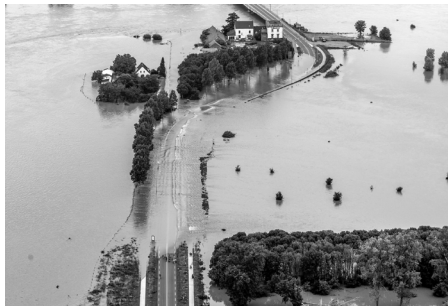
Figure 2.1.21. Photo of the highway during the flood in Maastricht Source: Google Images (2021)
