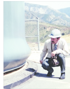
(b) Elephant foot buckling on a steel tank[59].
