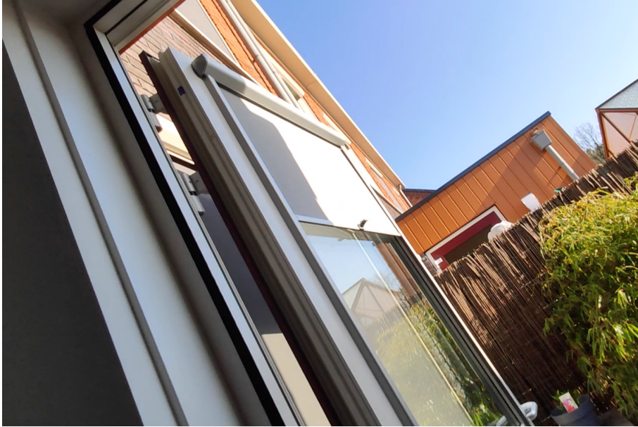
Figure 2.6. The retrofitted manual sunshade that can be drawn down to alter the light sensor readings.
