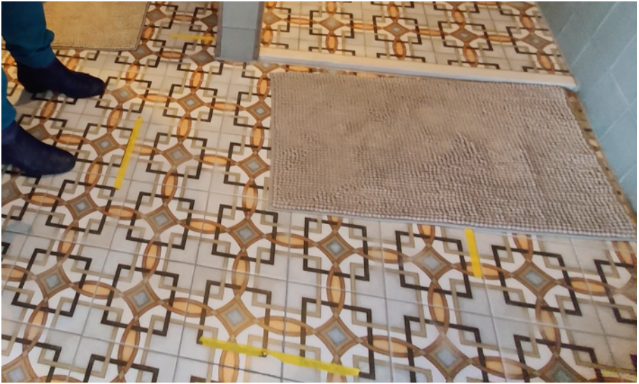
Figure 3.6. Ella's bathroom floor markings indicate where the floor gets warm and where it does not.
