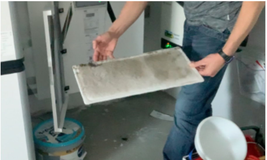
Figure 3.7. Gideon shows the dust that settles on the air filters.
