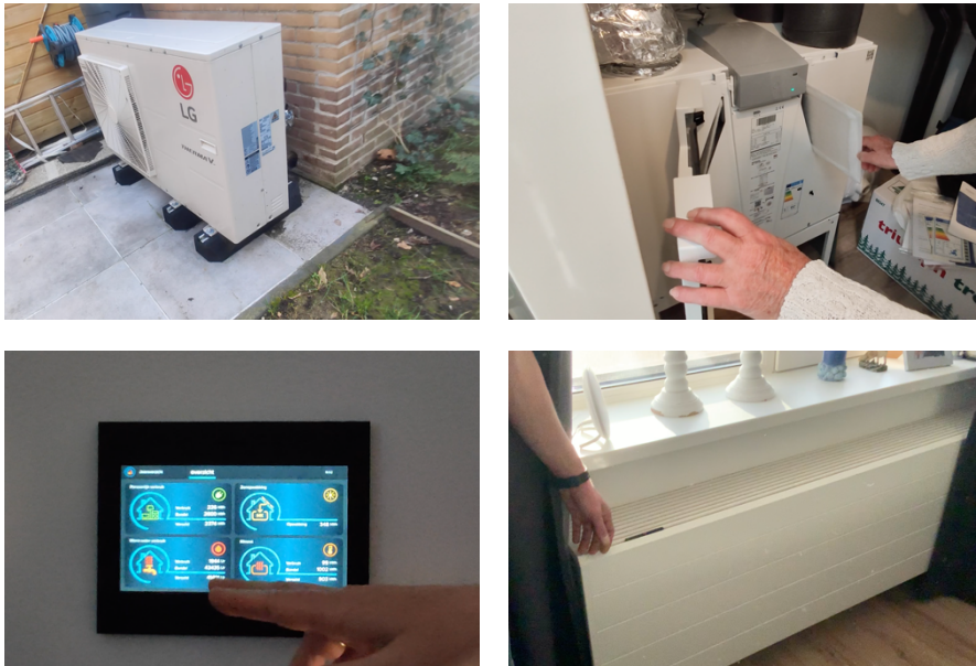
Figure 3.1. Technical features in the participating households (Left to right, top to bottom: an air-to-water heat pump, air filters being replaced, a display showing domestic hot water consumption and budget, low-temperature heating convectors)
